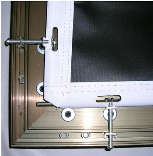
Place the fabric into the tensioning screws. Use a philips screw driver to tension all the screws and make sure the fabric is perfectly flat. **DO NOT OVER TENSION!**
